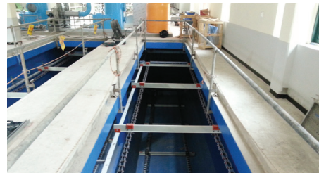
Sludge collector
